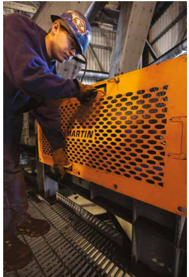
Guarding is one of the most common reasons for citations. All pinch points need well-designed guards to prevent access
